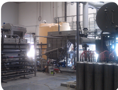
Waste water system during installation.
